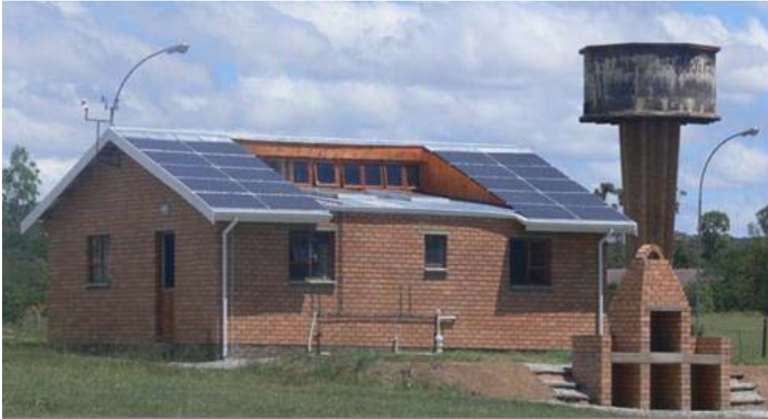
Figure 1: PV modules on the EEBIPV house [27]
